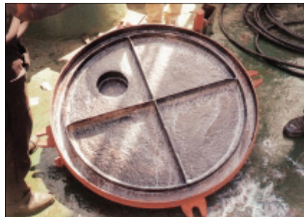
Step 5 Hatch cover surface immediately after RUST CONVERTER application.
