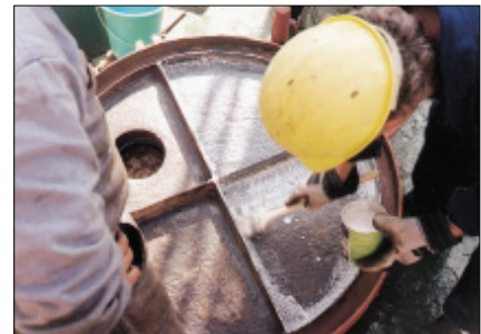
Step 3 Starting the application of RUST CONVERTER by brush or roller, depending of the surface structure.
