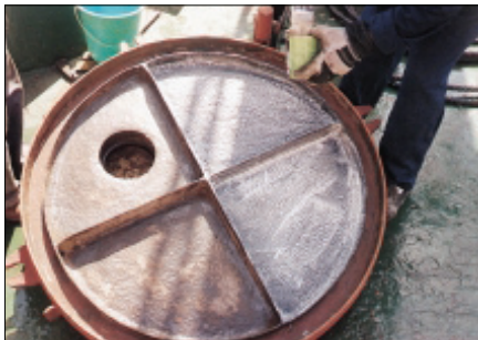
Step 4 Continuing RUST CONVERTER application.
