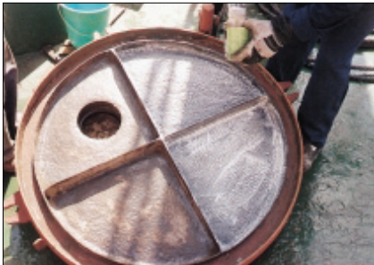
Step 4 Continuing RUST CONVERTER application.
