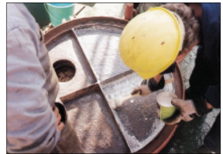
Step 3 Starting the application of RUST CONVERTER by brush or roller, depending of the surface structure.
