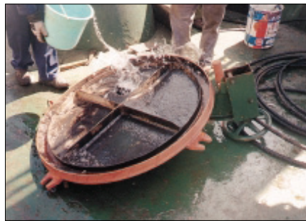
Step 2 Flushing with fresh water to remove atmospheric salts.
